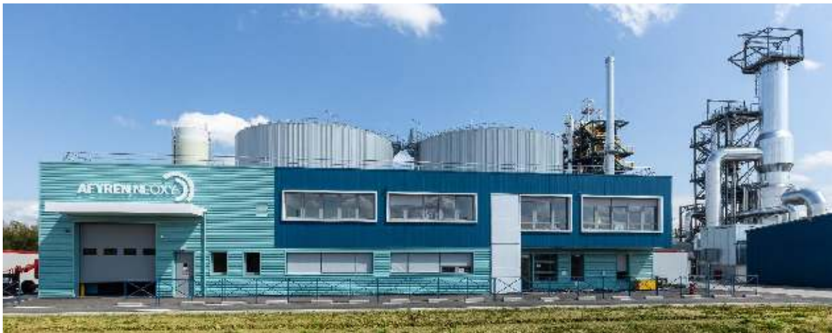
AFYREN NEOXY Plant
